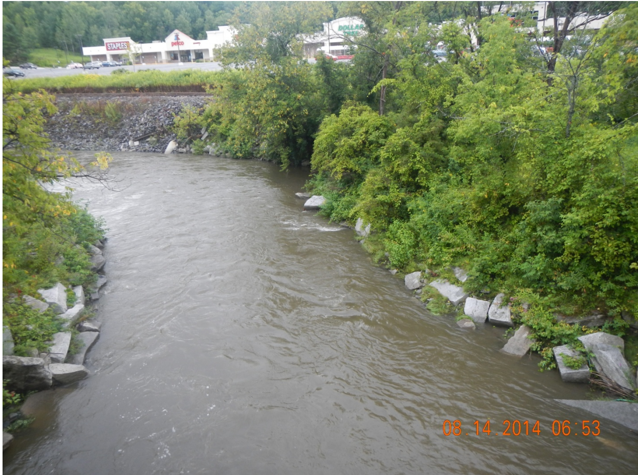
Figure 3: Stevens Branch, North side of the Bridge
